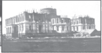
Capitol under construction — 1860-74
