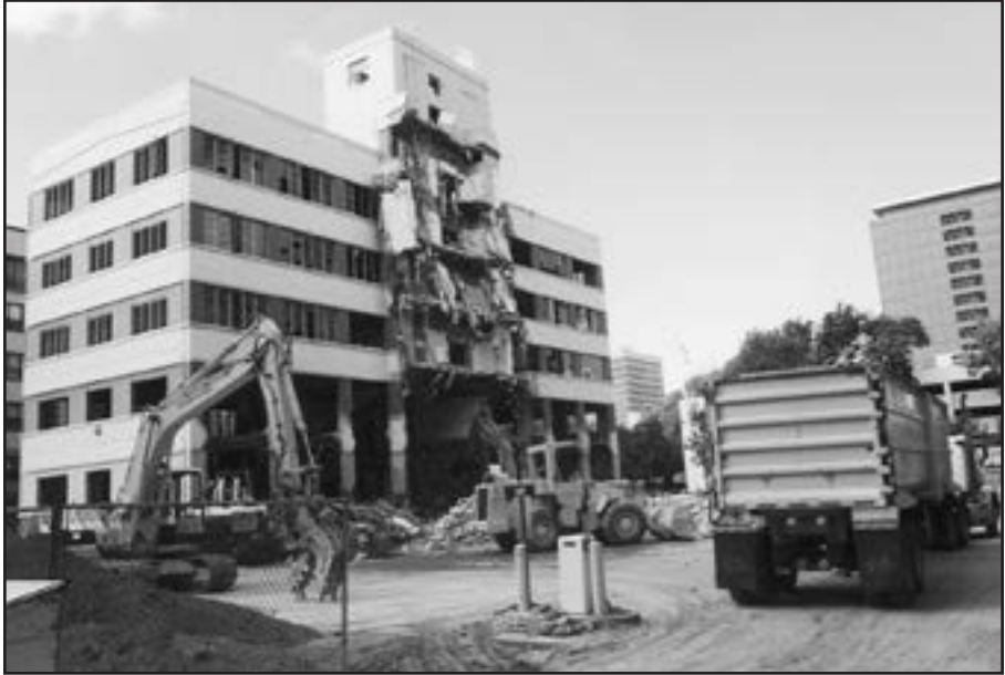
A portion of the LOB demolished during November 1999 remodeling
