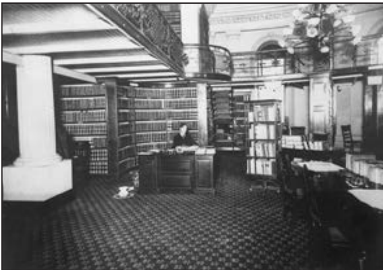
State Library, Law Department, 1904 (replaced Supreme Court Chambers in apse)
